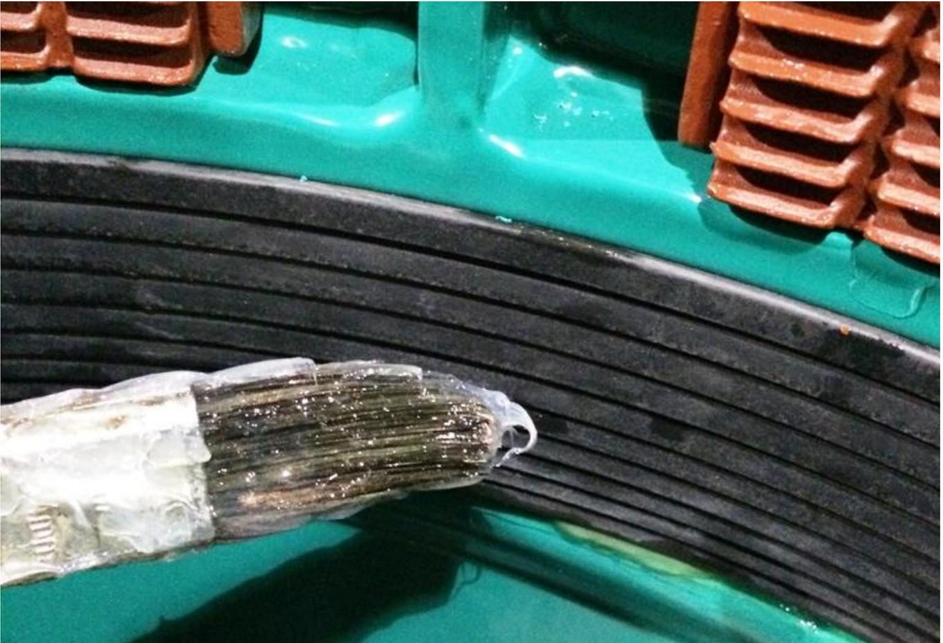
4. APPLY LOTS OF GASKET LUBRICANT – IF USED ON A POTABLE WATER LINE BE SURE TO USE A NSF CERTIFIED LUBRICANT!
